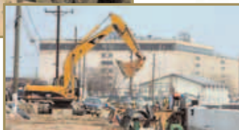
Left: Surcharging, an engineering process to raise the development area, is well underway.
