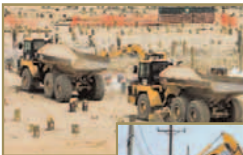
Left: Surcharging, an engineering process to raise the development area, is well underway.
